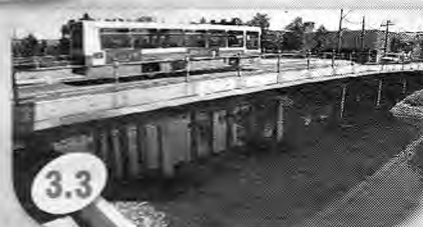
MACAULAY RD Repairs: Kensington Built: 1923 $680,000 to strengthen
