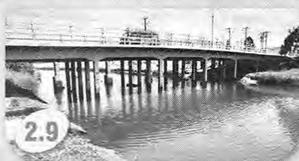
ARDEN ST Repairs: Nth Melbourne Built: 1923 $400,000 to strengthen
