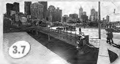
QUEENS BRIDGE Repairs: CBD Built: 1889 $405,000 to strengthen, repair steel and repaint
